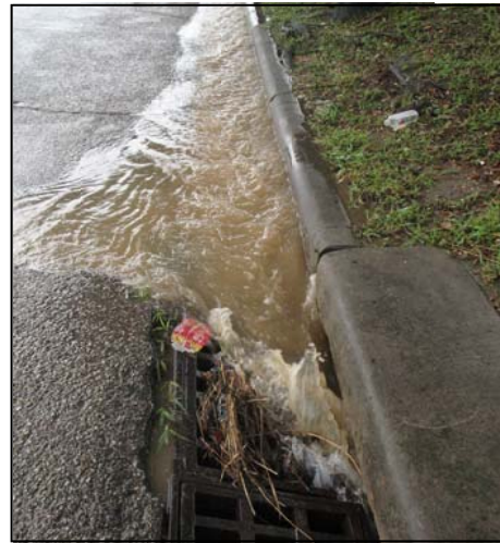
Stormwater running off an impervious surface. This water could be directed into a rain garden.
